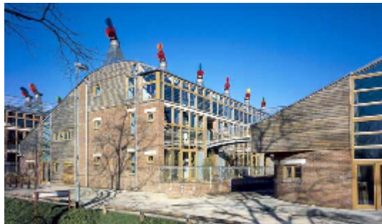
Figure 9 A view of the BedZED development
